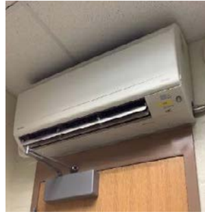
ECC Ductless Mini-Split System HP
