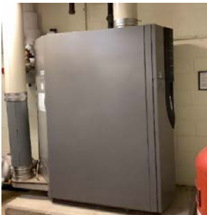
Condensing Boiler
