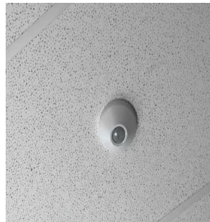
Ceiling Mounted Occupancy Sensor
