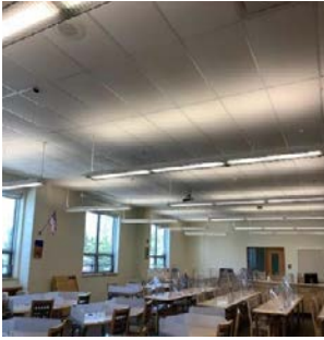
Media Center Pendent Mounted Lighting Fixtures
