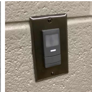
Wall Mounted Occupancy Sensor
